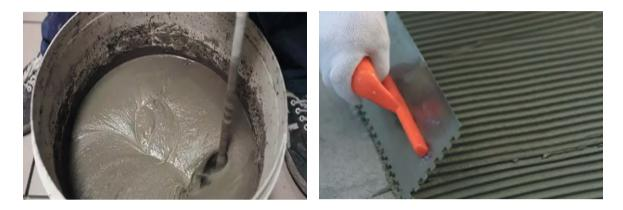
Fix the matting within the adhesive open time. Butt-join to the next matt, without overlaps. Leave 5-10mm gaps around the edge for substrate changes or movement joints.
