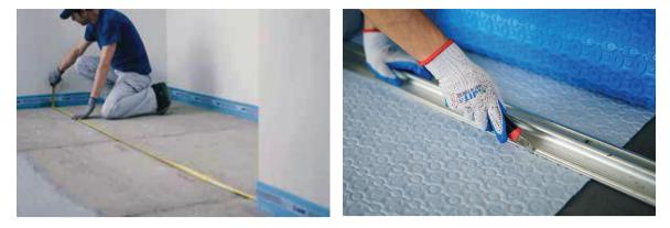
Lift matting and lay a bed of suitable tile adhesive using C2 grade or equivalent tile adhesive using 4mm notched trowel.
